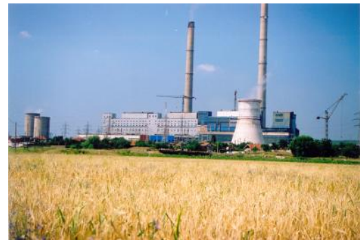
Craiova Power Plant
