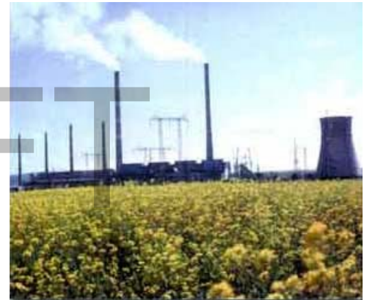
Maritsa East 2 Power Plant
